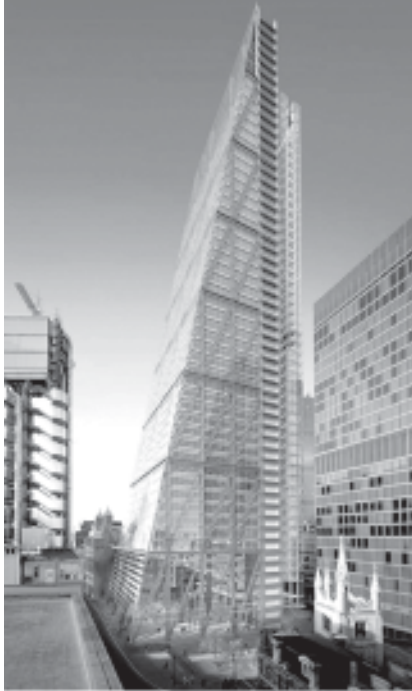
THE LEADENHALL BUILDING
